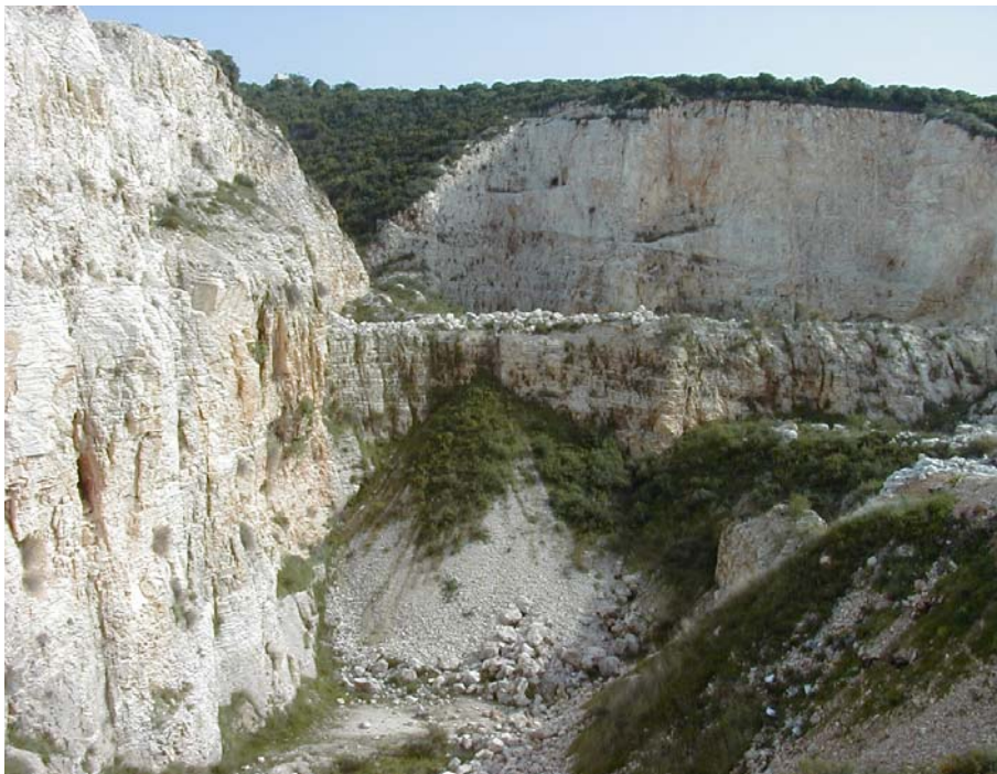
Figure 1. Three physiographical elements are present on a quarry site: the cliffs, the platforms and the embankments.
