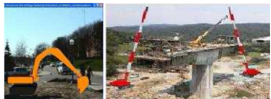
Figure 13: Example of augmented construction view [3]
