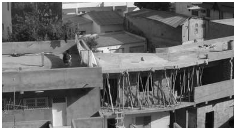
Fig. 1. Construction of new buildings in Dakar.
