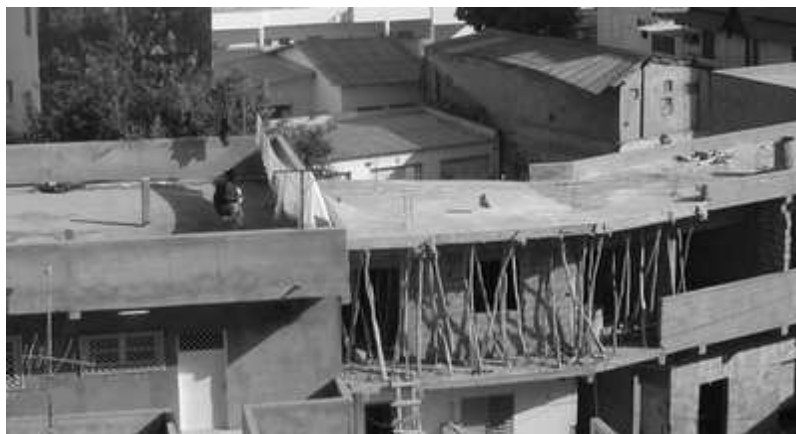
Fig. 1. Construction of new buildings in Dakar.
