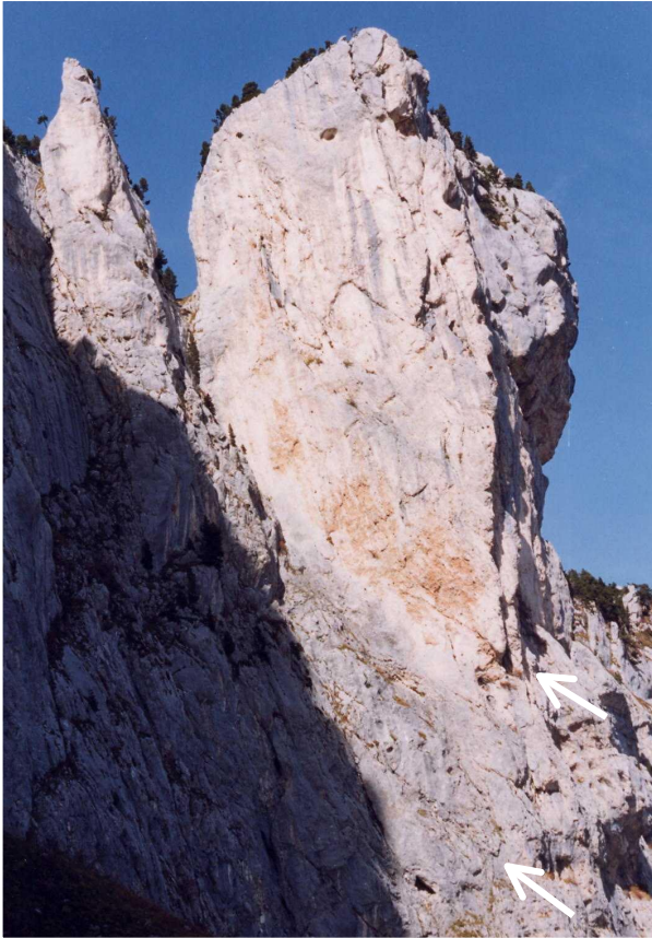
Fig. 2. Example of a potential rock slide in Grenoble area (height: 130 m; volume: 350 000 m 3 ); potential sliding planes are shown by the arrows. Smaller potential rock falls are visible on the upper right (overhangs).
