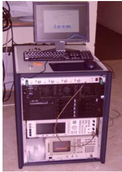
Figure 3: Receiving and acquisition system.
