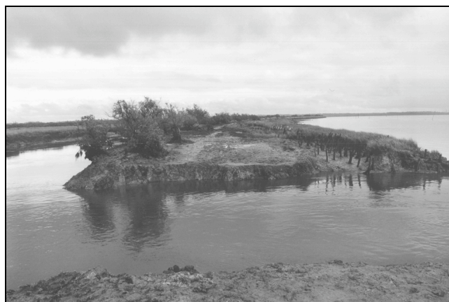
Figure 4: Accidental breach in the Graveyron-polder sea dike. From right to left in the background: Arcachon Bay (F), the still eroding sea dike and part of a growing saltmarsh (figure 2c).
