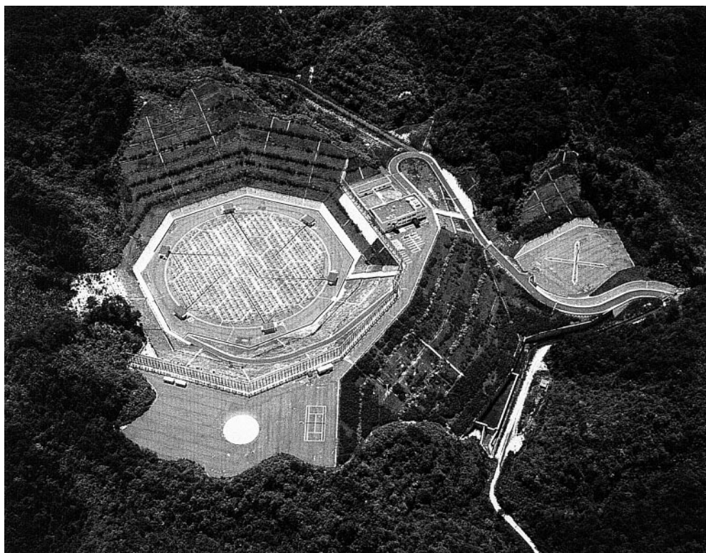
Fig. 6. An aerial view of the MU radar near Shigaraki, Japan
