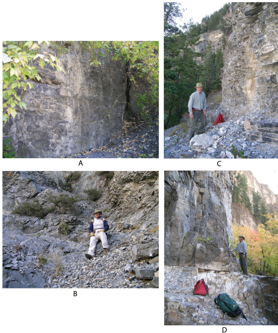
Fig. 7. Examples of Q measurement sites (see Fig. 2 for locations). (A) Site Q13 on a shallowly-dipping fold limb, width of exposure shown is about 3 m, Q=4.10 , relative block size =6.83 , estimated friction angle =72^\circ , rock tightness =0.20 , roughness of discontinuities =3 , number of discontinuities =10 . (B) Site Q23 on a steeply-dipping fold limb, see geologist for scale, Q=0.19 , relative block size =0.67 , estimated friction angle =45^\circ , rock tightness =0.29 , roughness of discontinuities =1 , number of discontinuities =32 . (C) Site Q8 in the hinge zone of a gentle fold, see geologist for scale, Q=0.14 , relative block size =0.57 , estimated friction angle =45^\circ , rock tightness =0.25 , roughness of discontinuities =1 , number of discontinuities =100 . (D) Site Q12 on a shallow-dipping limb, see geologist and backpacks for scale, Q=1.72 , relative block size =2.75 , estimated friction angle =68^\circ , rock tightness =0.25 , roughness of discontinuities =2.5 , number of discontinuities =24 .
