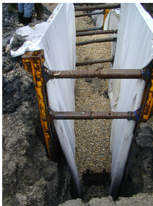
Fig. 13. Detail of deep drain trenches.
