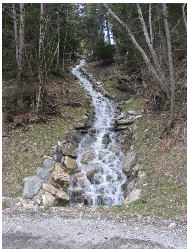
Fig. 11. Detail of the surface dewatering system on the stable grounds above the panoramic road – channel with a longitudinal slope of around 30%, protected with rip rap.
