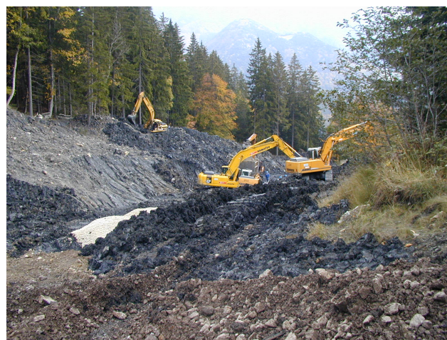
Fig. 12. Execution of deep drain trenches.
