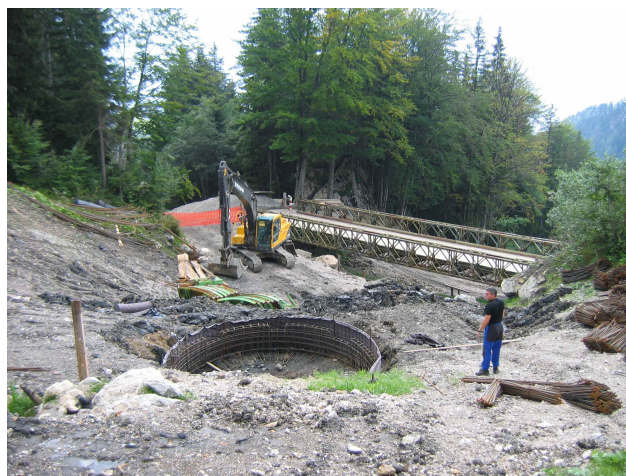
Fig. 16. Execution of a RC well just above the pontoon bridge.
