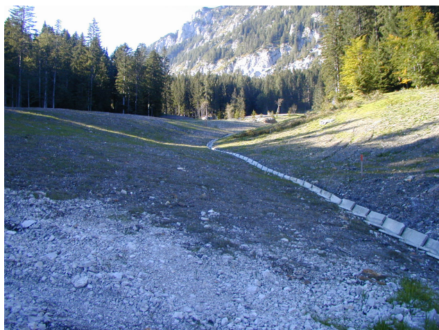
Fig. 15. Stabilised part of the Macesnik landslide above the pontoon bridge by introducing several deep drainages and peripheral and central surface drainage.
