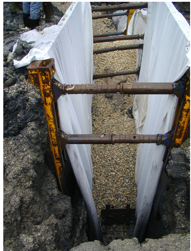
Fig. 13. Detail of deep drain trenches.
