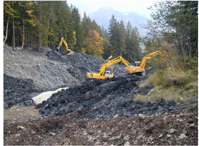
Fig. 12. Execution of deep drain trenches.
