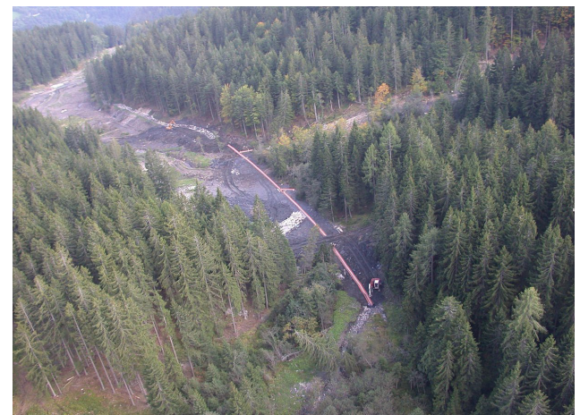
Fig. 10. Executed peripheral surface drainage at the western landslide edge above the prefabricated bridge.
