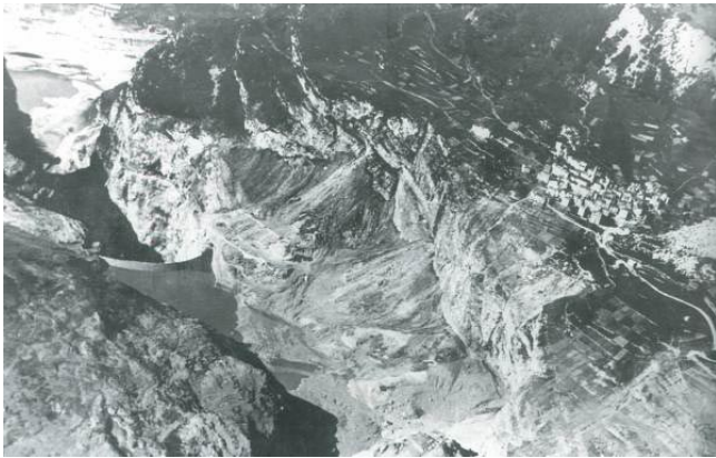
Fig. 12. The Vajont valley just after 9 October 1963, landslide event. In the left part of the picture it is possible to see the Vajont dam, as it is now, which was not damaged by the overtopping water.
