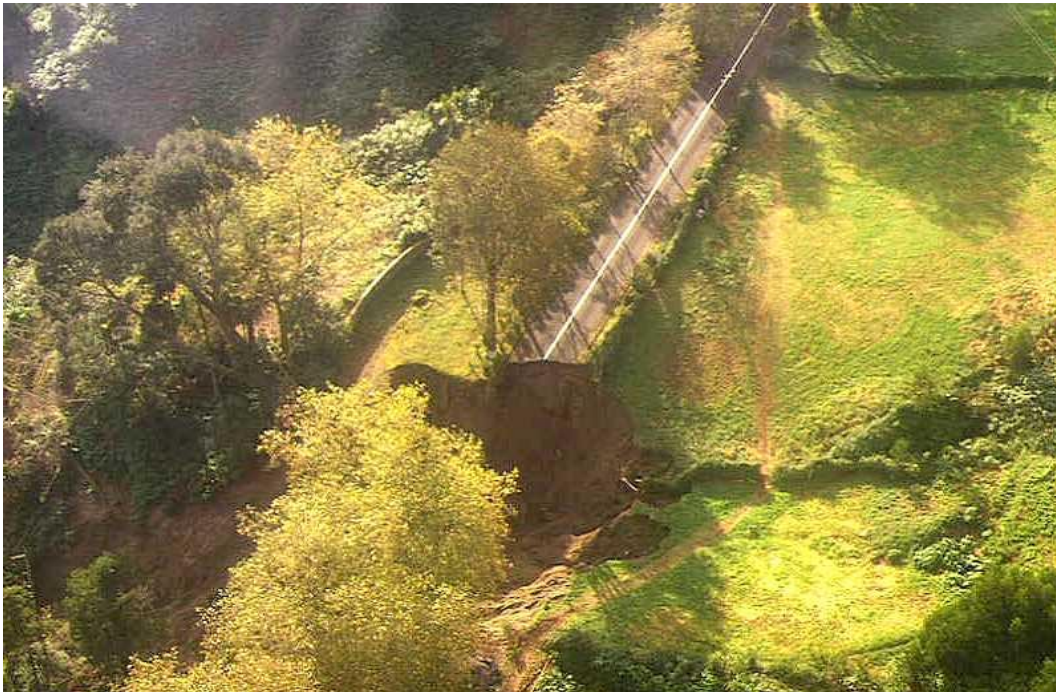
Fig. 7. Road cut by the collapse of the edge of a streamline at Furnas Volcano, during the 1997 Ribeira Quente event.
