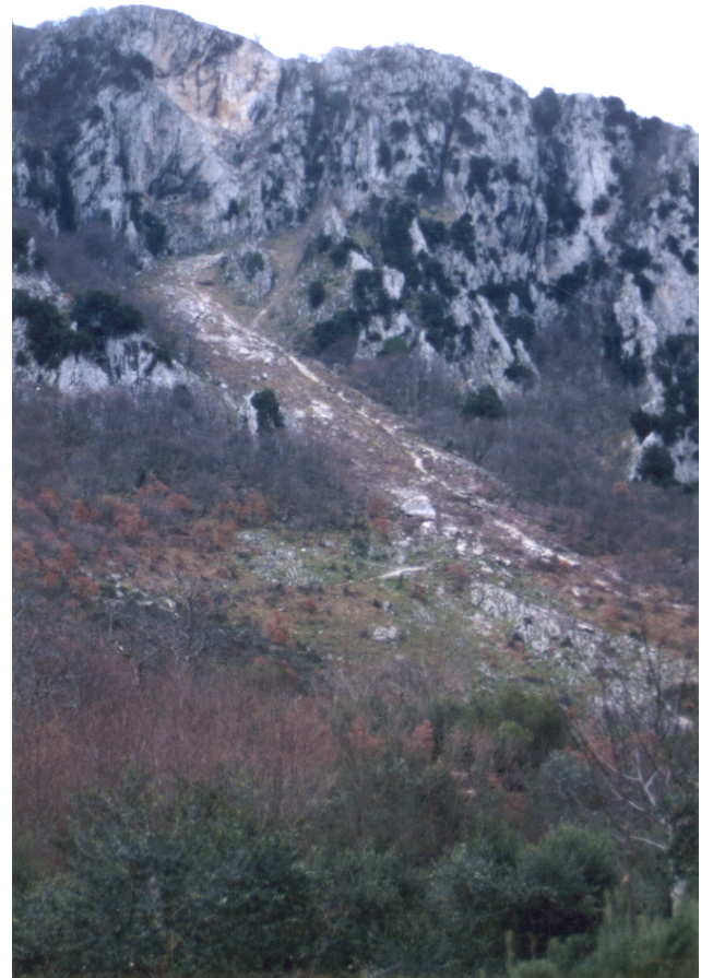
Fig. 5. Rock-fall source area in the mountain above the town of Valva. Note the high gradient of the talus slope, and the freshness along the rock-fall path, the latter testifying to recent slope movement activity.
