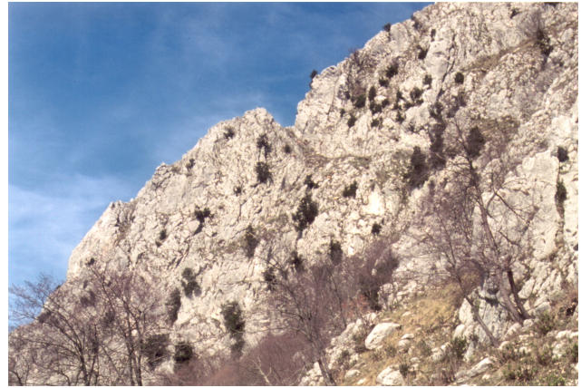
Fig. 7. View of the western slope of Mt. Marzano: the two main discontinuity systems that are present in this portion of the mountain make likely detachment as wedge failures in the carbonate rocks.
