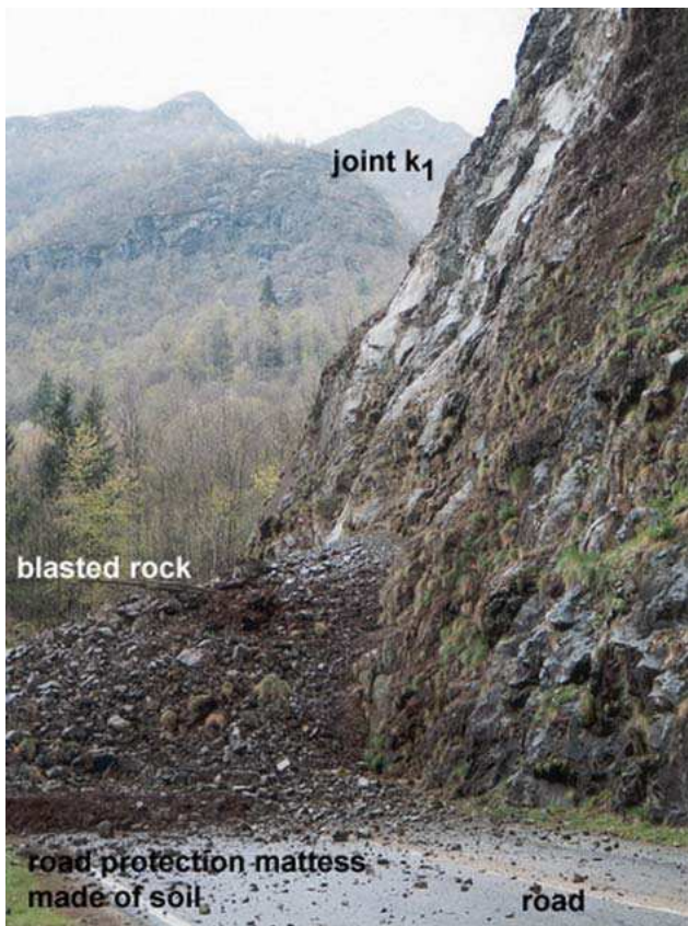
Fig. 6. Result of the blast. It is possible to see the joint k_1 that was behind volume n. 1 and the good fragmentation of the blasted rock.
