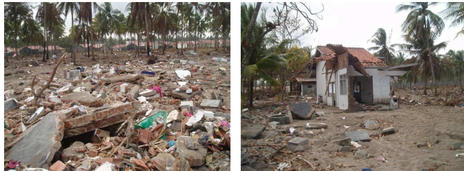
Fig. 12. The remains of traditional brick houses after inundation to a depth of ca. 3 m (a). There were a few partially intact (b).
