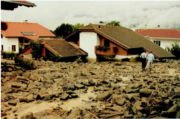
Fig. 2. The debris flow event of 16 August 1997 damaged buildings situated on the Wartschenbach fan, community of Nußdorf-Debant, Austria.
