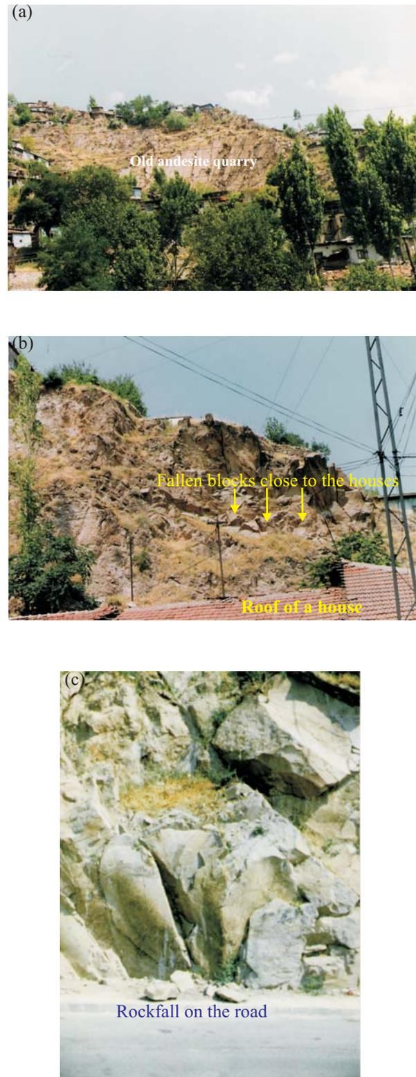
**Fig. 2.** (a) General view of the Timurlenk Hill and an old andesite quarry, (b) fallen blocks threatening a house, (c) rockfall on a road.
