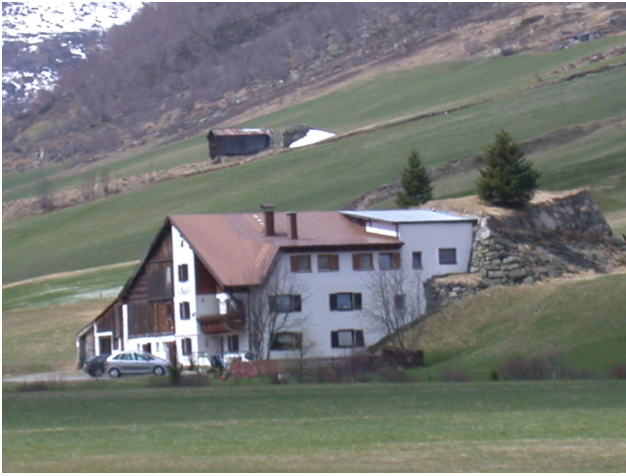
Fig. 3. Building with an integrated avalanche deflector on the uphill side of a building located in the community of Galtür.
