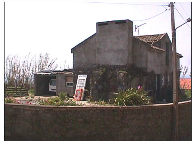
Fig. 9. Dwelling with external walls both in stone and in concrete blocks.
