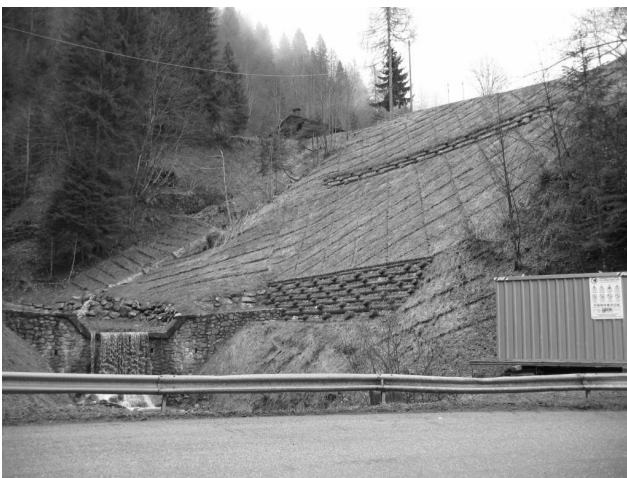
Fig. 8. Lower part of the “La Maina” landslide after the consolidation.
