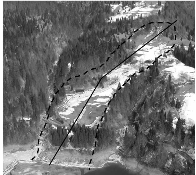
Fig. 2. The “La Maina” landslide. Modelling cross section is highlighted.
