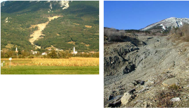
Fig. 4. A far and a close view of the Slano Blato landslide.
