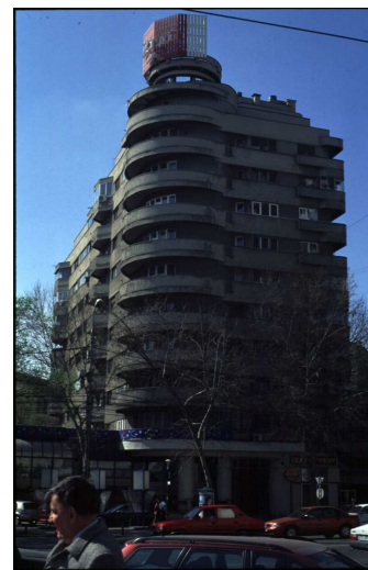
Fig. 7. Examples of post-1977-Vrancea-earthquake buildings in Bucharest (a) without changed conformation after retrofit ("Pherekyde"); (b) with changed conformation after retrofit ("Turist"); (c) replacing those collapsed ("Dunărea").
