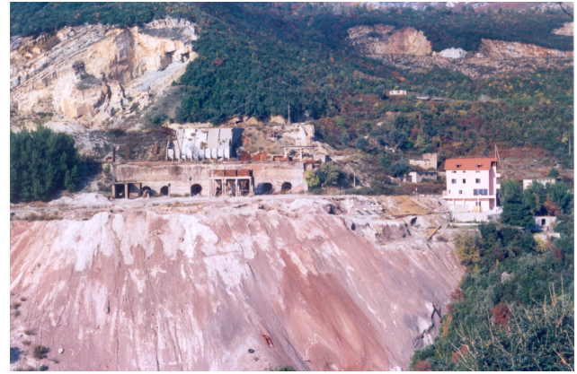
Fig. 9. Quarry facilities which were active during the Communist period for lime production from limestones of Burdigalian age. The quarry is located close to the village of Linxe, in the Dajt province, just east from Tirana. Wastes from the activity were discharged in the Tirana river, running just below, and some of its main tributaries.
