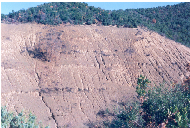
Fig. 6. Slope in the Gramsh area, south of Elbasan: the slope in flysch deposits, originally covered by vegetation, was used for agriculture practice, with the farm tractors working along the steepest slope gradient. This resulted in development of rills and gullies, which in turn forced the farmers to abandon the slope.
