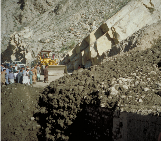
Fig. 1. Debris flow that occurred during sunny weather in June 1997 on the Karakoram Highway, Pakistan. This debris flow lasted approximately 2 h in the early afternoon and included several surges. The lack of rainfall allows us to suppose that this event was triggered by intense snowmelt.
