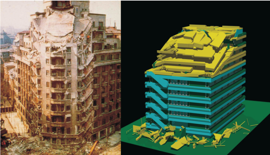
Fig. 4. Multi layer collapse of the upper stories: in reality (Münchener Rück, 1996) and as simulation.
