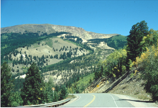
Fig. 3. View of the Slumgullion landslide, taken uphill from the State Highway 149.
