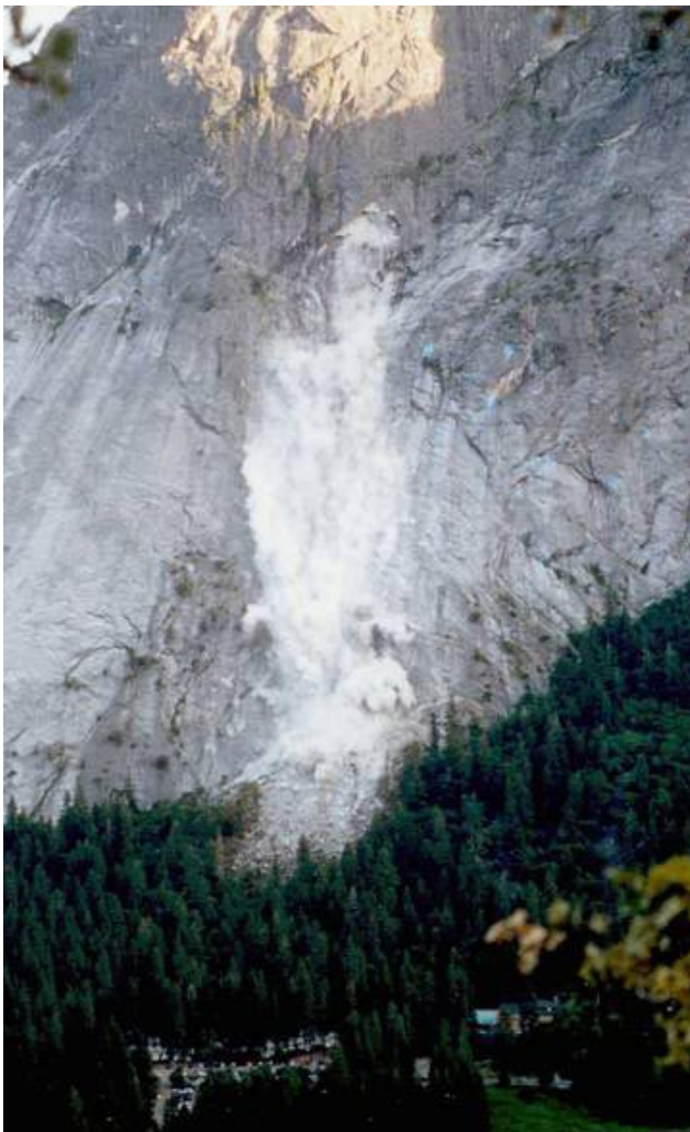
Fig. 2. Rock fall on 13 June 1999 above Curry Village, Yosemite Valley, California. The failure involved 213.4 \text{ m}^3 of granitic rock. Photograph by Lloyd De Forrest (used with permission).
