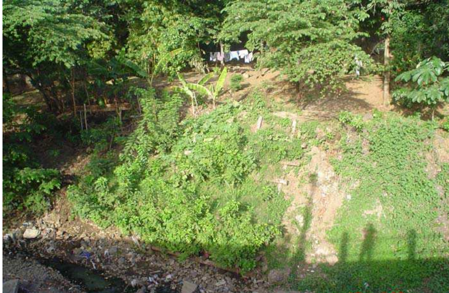
Fig. 8. The riverbank protection, 7 months after cuttings planted.
