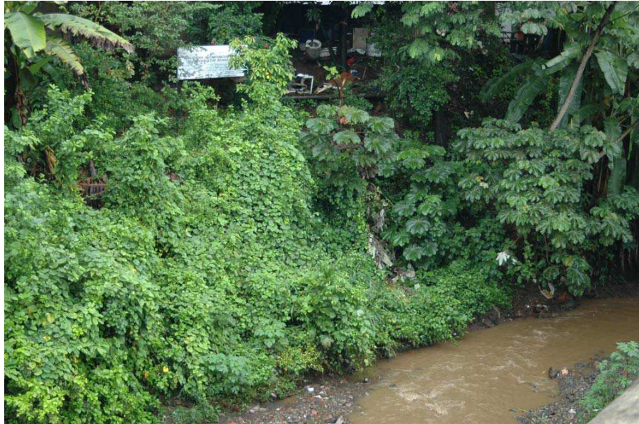
Fig. 10. The riverbank protection, 44 months after cuttings planted.
