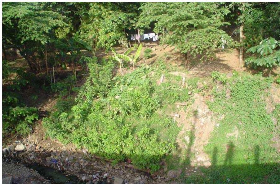
Fig. 8. The riverbank protection, 7 months after cuttings planted.
