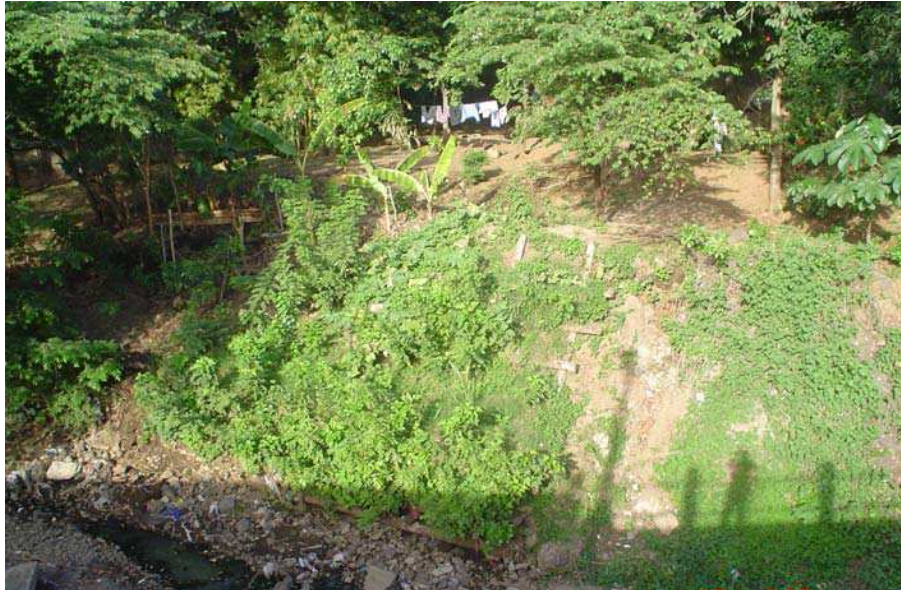
Fig. 8. The riverbank protection, 7 months after cuttings planted.
