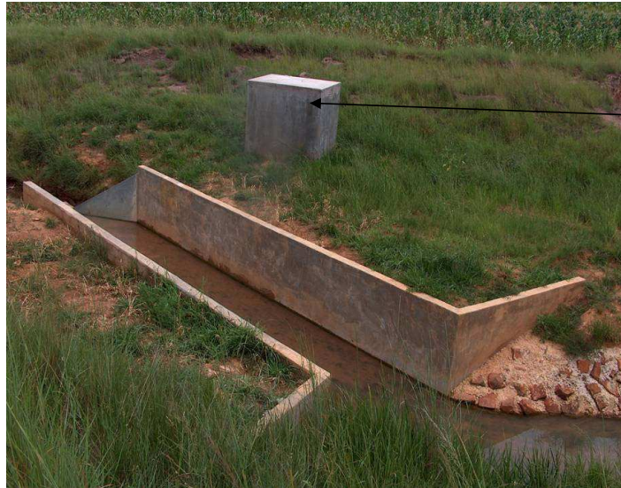
Fig. 4. An operational H-Flume in the Potshini catchment.
