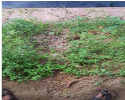
Fig. 8. CP-less density, non uniform vegetation with soil erosion, after 7 months.
