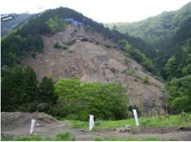
Fig. 5. General view of the landslide site (14 May 2006).
