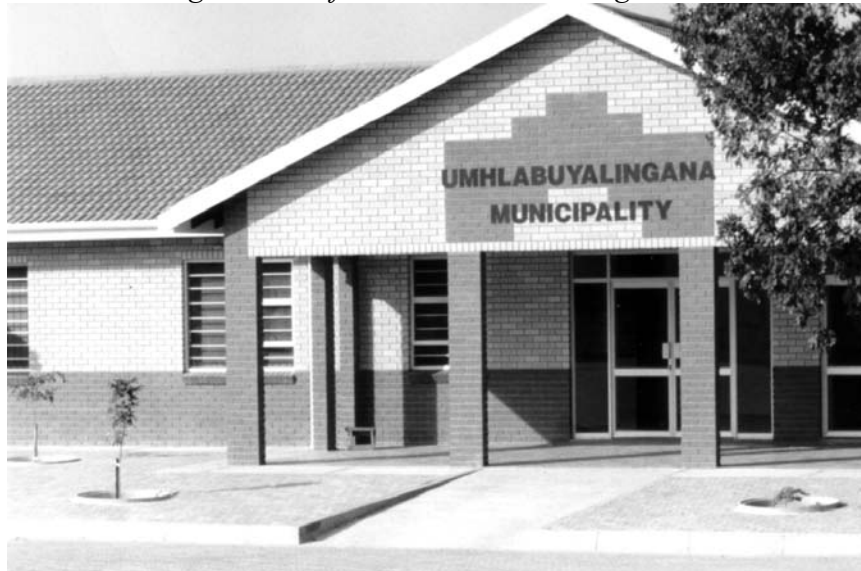
Figure 13: New municipal buildings
