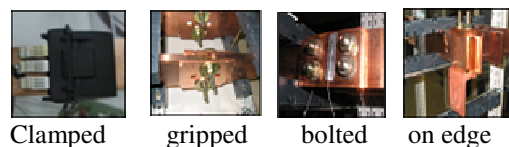
Fig 3 Different types of electrical joints.
