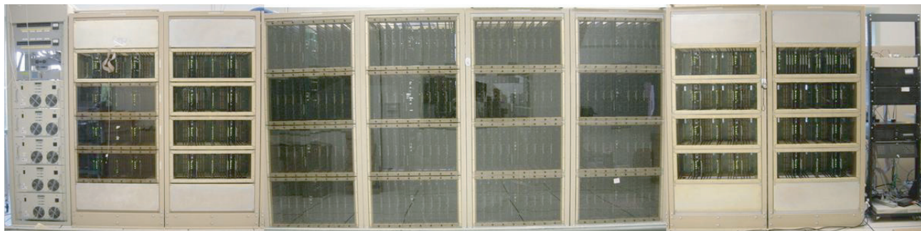
Fig. 1. ALMA Correlator under construction (first quadrant).
