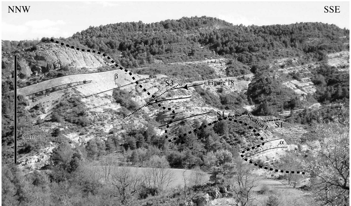
Figure 12 : Section I outcrop, located on Figure 11. Dipmeter measurements follow the dashed line ; the lowest part of the section is not visible on this picture. The main sliding surfaces S1 and S3 are underlined, together with stratigraphic markers \alpha and \beta (Figure 15). View to the south east.
