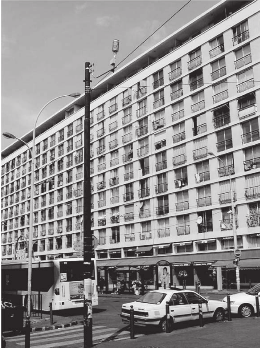
Figure 11. Example of a shielded T-RH sensor assembly at a site in the city centre.
