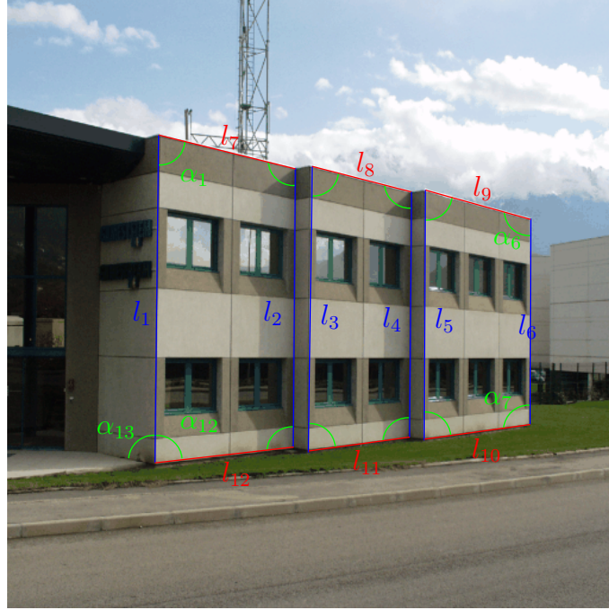
Figure 18: Metric quality measures on the reconstruction for the BUILDING dataset. The segments with same color should have equal length and the angles should be \pi/2 .
