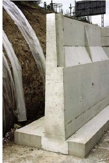
FIGURE 4.2 – Mur cantilever.
