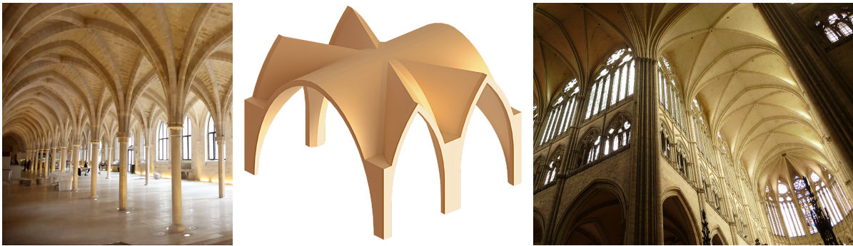
Figure 7.38: Different types of rib vaults. From the left: quadripartite vault of the Collège des Bernardins , Paris, scheme of a sexpartite vault, barlong vaults of the Cathedral of Amiens.
