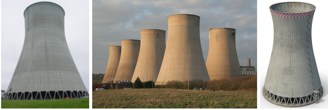
Figure 7.32: Cooling towers in the form of hyperbolic hyperboloids.
